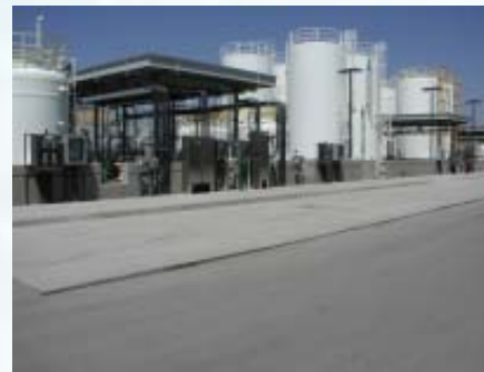
Chemical Loading Area
