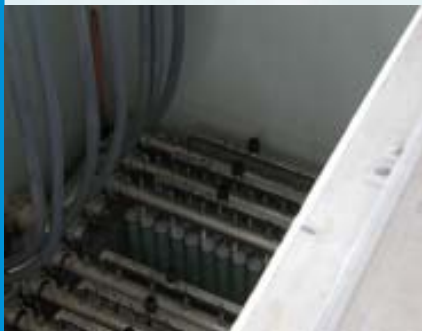
AWPF Microfiltration - Rack Installed in a cell
