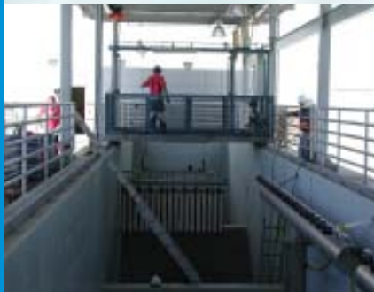
AWPF Microfiltration - Rack Lowered into a cell
