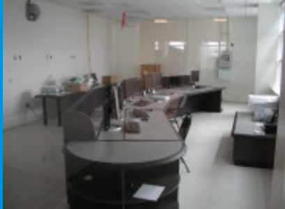
AWPF Control Room
