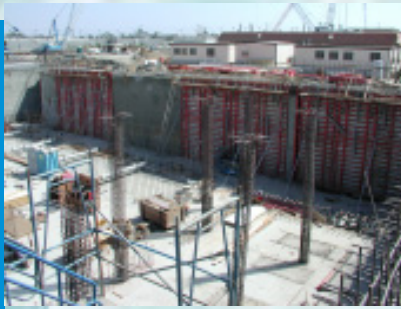
AWPF Microfiltration West Side Exterior Walls
