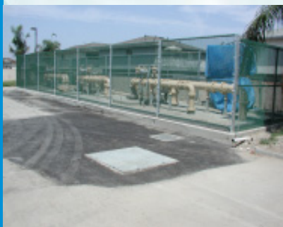
Barrier Well Site I-31
